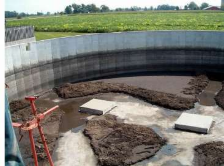
Manure storage tank
