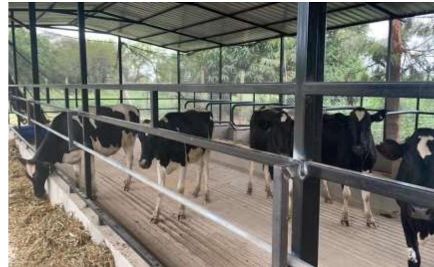
Shading by providing roofing and net suspension
