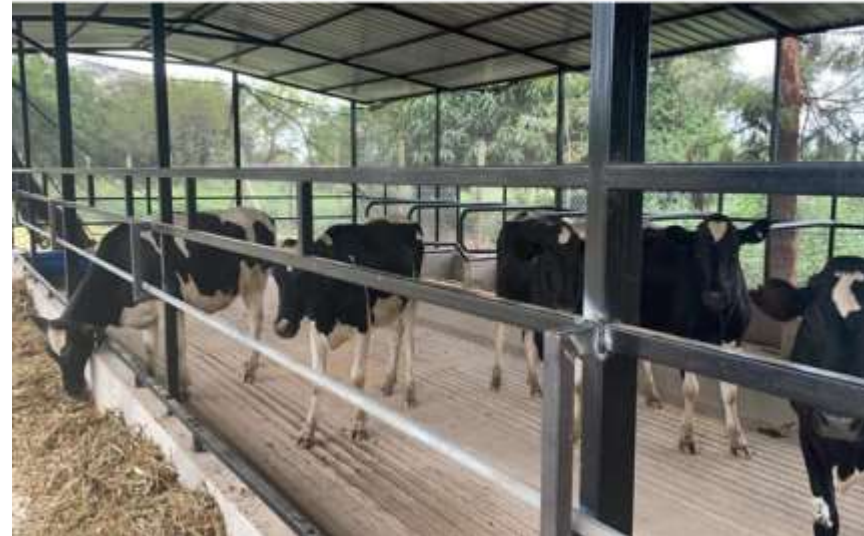
Shading by providing roofing and net suspension
