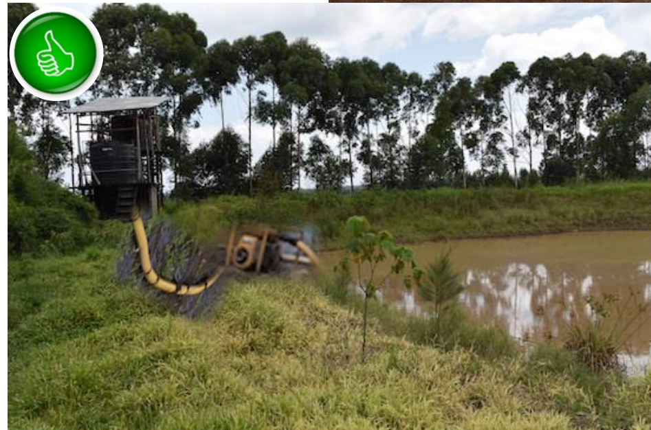
Water pumped to overhead tank
