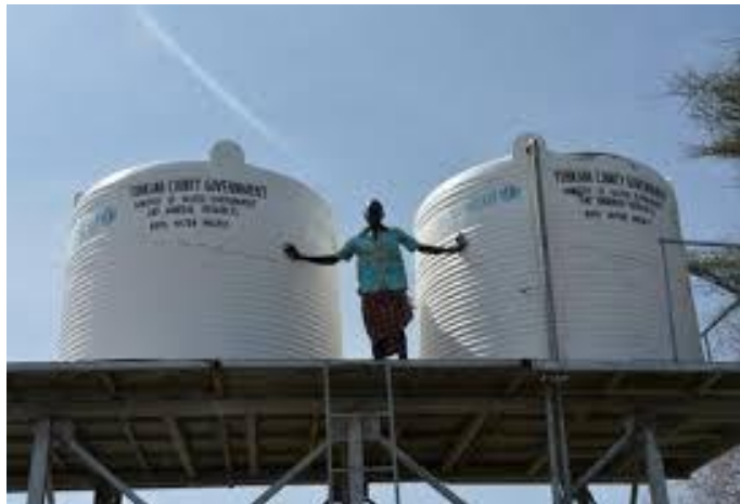
Elevated plastic tanks
